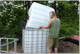
Upper IBC(floating drum): Lift the second IBC out of its metal cage. Open one side of the container for the water in/outlet. Cut it also a bit shorter (-3") to fit better into the lower IBC. Test if the upper IBC slides into the lower IBC easily. If you still feel tension cut a little more of the sides.
