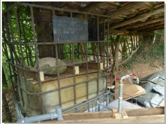
Use a palette on top of the upper IBC. Give some weight, with sand bags or stones to have some pressure in the gas storage. 10Kg on 1m<sup>2</sup> give you 1mbar; 150kg/m<sup>2</sup>=15mbar, that's a good pressure!
