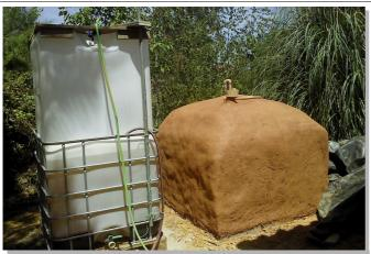
Fill the lower IBC with water and let the upper tank emerge into it. Stop in the middle and test if he keeps the pressure for 1day, to be sure it is gas tide.
