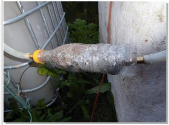
Connect the gas outlet of the digester with the in/outlet of the floating drum.
