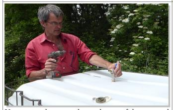
Now create the gas outlet on the top of the emerged IBC. Connect the bulkhead and the valve. Make sure everything is airtight.
